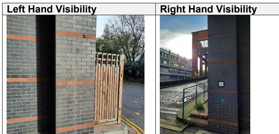
The northern access junction (egress) has been designed as the site egress with a no-entry sign and the building line angled to allow right hand visibility towards Observatory Car Park. A fence appears to have been erected which may need to be removed to allow suitable visibility.
